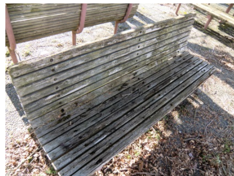
Fig. 3 Wooden benches decayed
